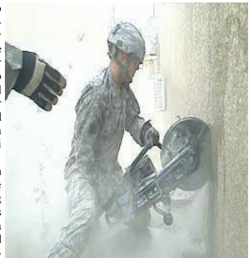
Cpl. William Watson, native of Kimball, MI, cuts masonry wall for the frame of the rear door of building #3.
