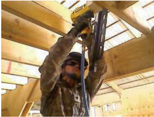
Spc. Ian Farnes, a native of Laural, MT, nails a ceiling joist in place on the second floor of build #3.
