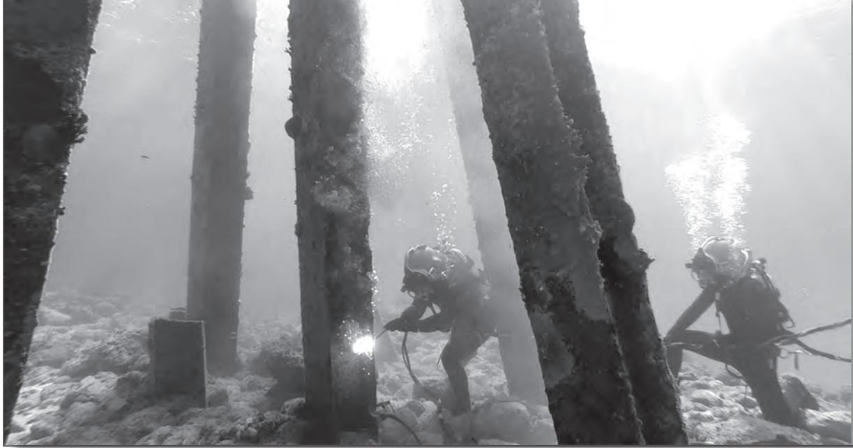
**The lead salvage diver uses a BROCO exothermic cutting torch to detach a center I beam from an ATON while a second-class diver tends to the lead diver, Andros Island, Bahamas.**
