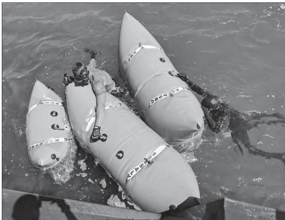
**Second-class divers prepare to deflate lift bags after successfully relocating the attached I beams to the pier, Andros Island, Bahamas.**
