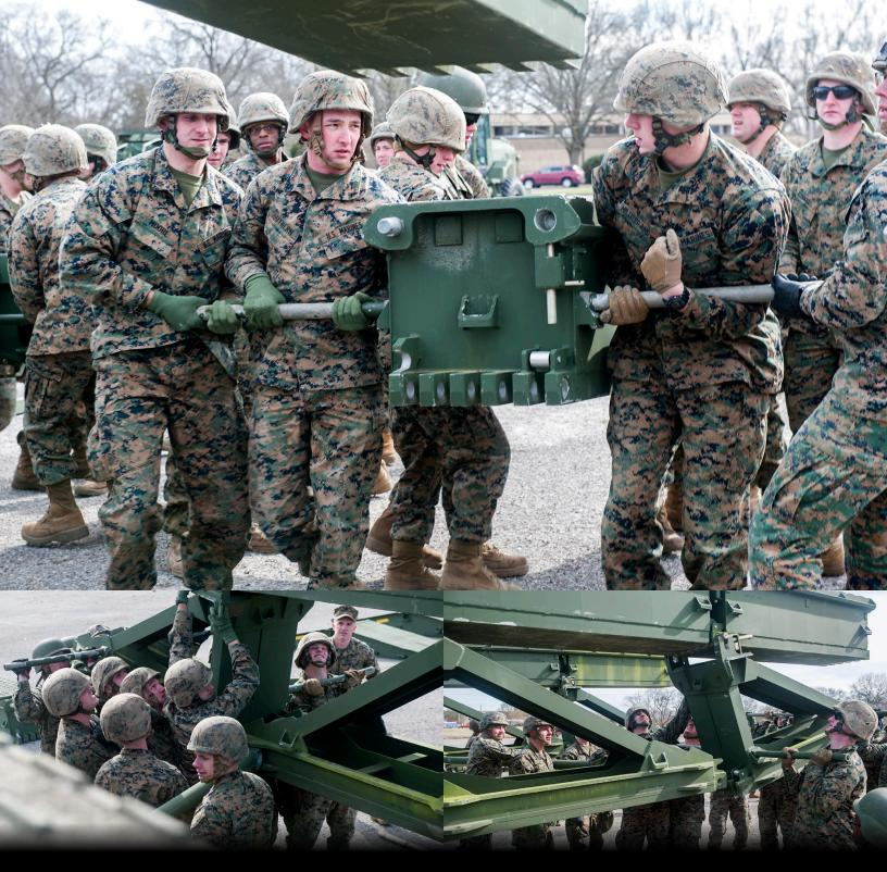
MILLINGTON, Tenn. (Feb. 8, 2019) Marines assigned to Bridge Company C, 6th Engineer Support Battalion, based in Millington, conducts improved ribbon bridging operations at Naval Support Activity Mid-South to provide essential training that enhances military readiness. Bridge Company C falls under the command of 4th Marine Logistics Group, Marine Forces Reserve.
