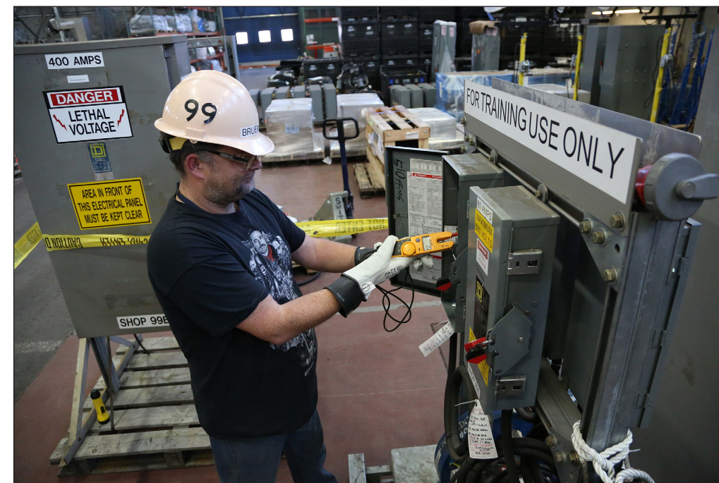
Rodney Breummer, a temporary services electrician with Shop 99, uses a volt meter to confirm a device has been properly powered down during a lock-out tag-plus procedure demonstration in Building 462, Feb. 25, at Puget Sound Naval Shipyard & Intermediate Maintenance Facility. (PSNS & IMF photo by Max Maxfield)
