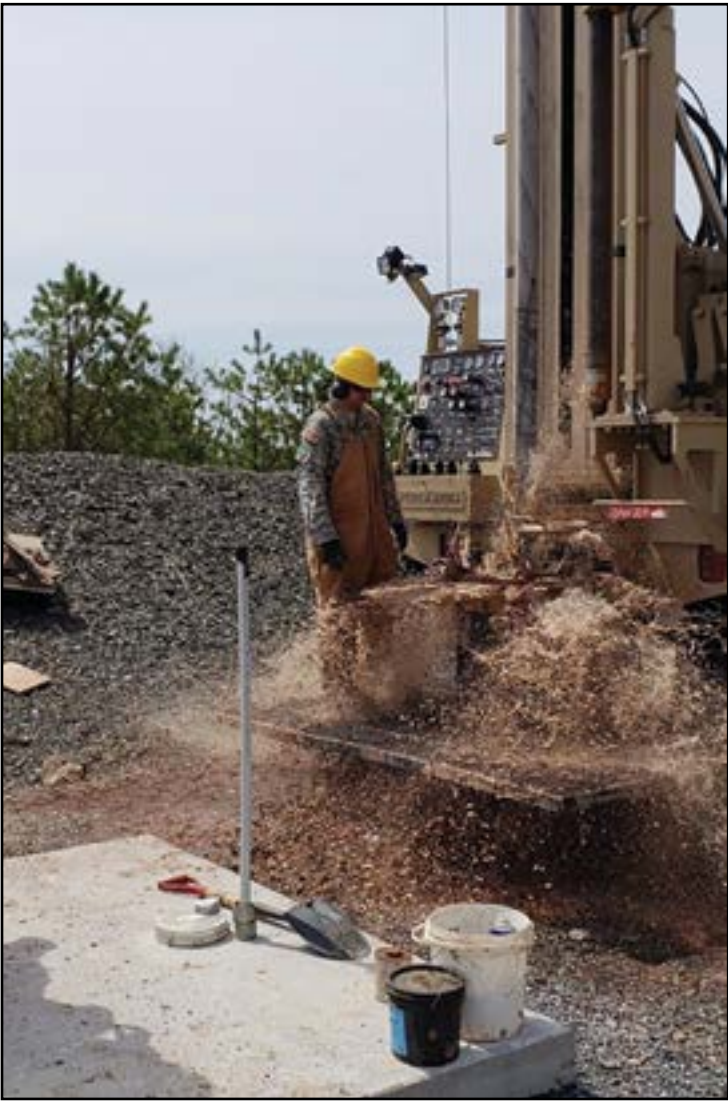
Above: A Soldier assigned to the 247th Engineer Detachment conducts drilling operations at Fort Indiantown Gap, Pennsylvania, during the unit's annual training in the spring of 2018. The unit spent their AT at FIG drilling a 500-foot well to be used for fire suppression in support of FIG rage control and a 100-foot well for ground water monitoring. The 247th has completed their AT at FIG each of the past four years, completing similar projects. (Photo by Staff Sgt. Steve London, Training NCO, 248th Engineer Company)
