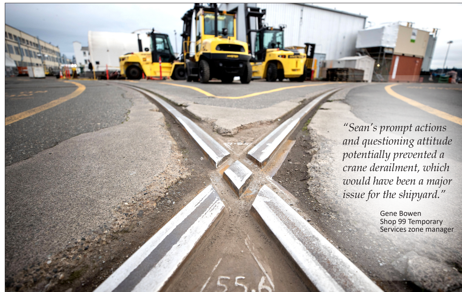
A repaired diamond-shaped crane track junction, more commonly known as a track "frog," near the end of pier six was recently repaired, thanks to the quick eye of shipyard employee Sean Davenport, a pipefitter supervisor with Shop 99 Temporary Services. (PSNS & IMF photo by Scott Hansen)
