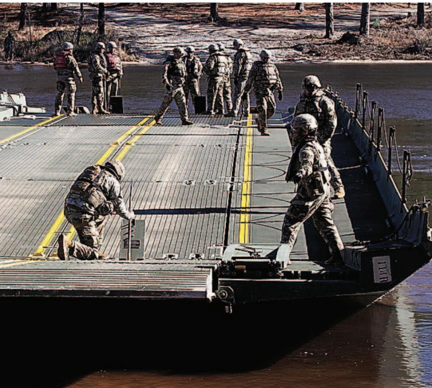
Soldiers from 1st BCT, 82nd Abn. Div. and the 502nd Multi-Role Bridge Co., 19th Engr. Bn. work together to conduct final checks on the connection of a ribbon bridge during a wet gap crossing exercise at MacArthur Lake, Jan. 9. This is to ensure safety of the vehicles and Soldiers during the crossing.
