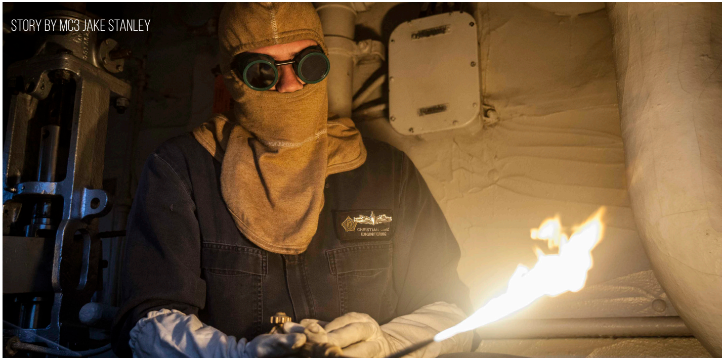
Navy Hull Technician Second Class Christian Cruz adjusts the oxidizing flame of a torch tip.
