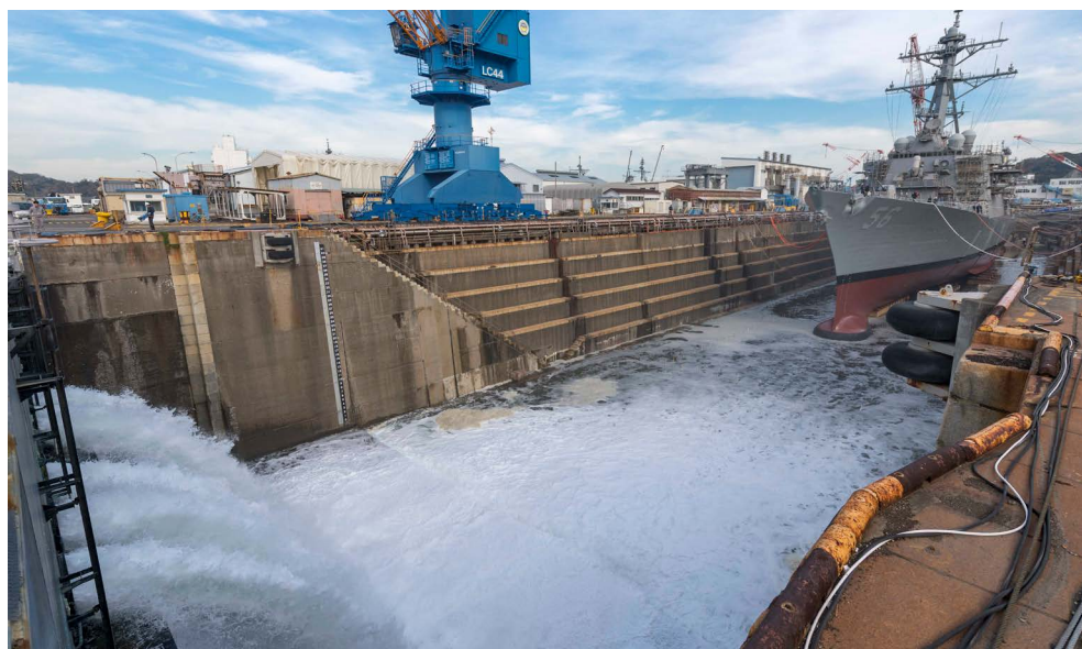
The Arleigh Burke-class guided missile destroyer USS John S. McCain (DDG 56) prepares to undock as a dry dock is flooded in order to test the ship's integrity. McCain is departing the dock after an extensive maintenance period in order to sustain the ship's ability to serve as a forward-deployed asset in the U.S. 7th Fleet area of operations. (U.S. Navy photo by Mass Communication Specialist 2nd Class Jeremy Graham/Released)
