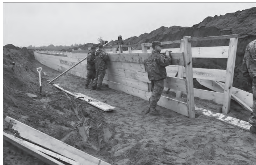
Sappers constructing the retaining wall.
