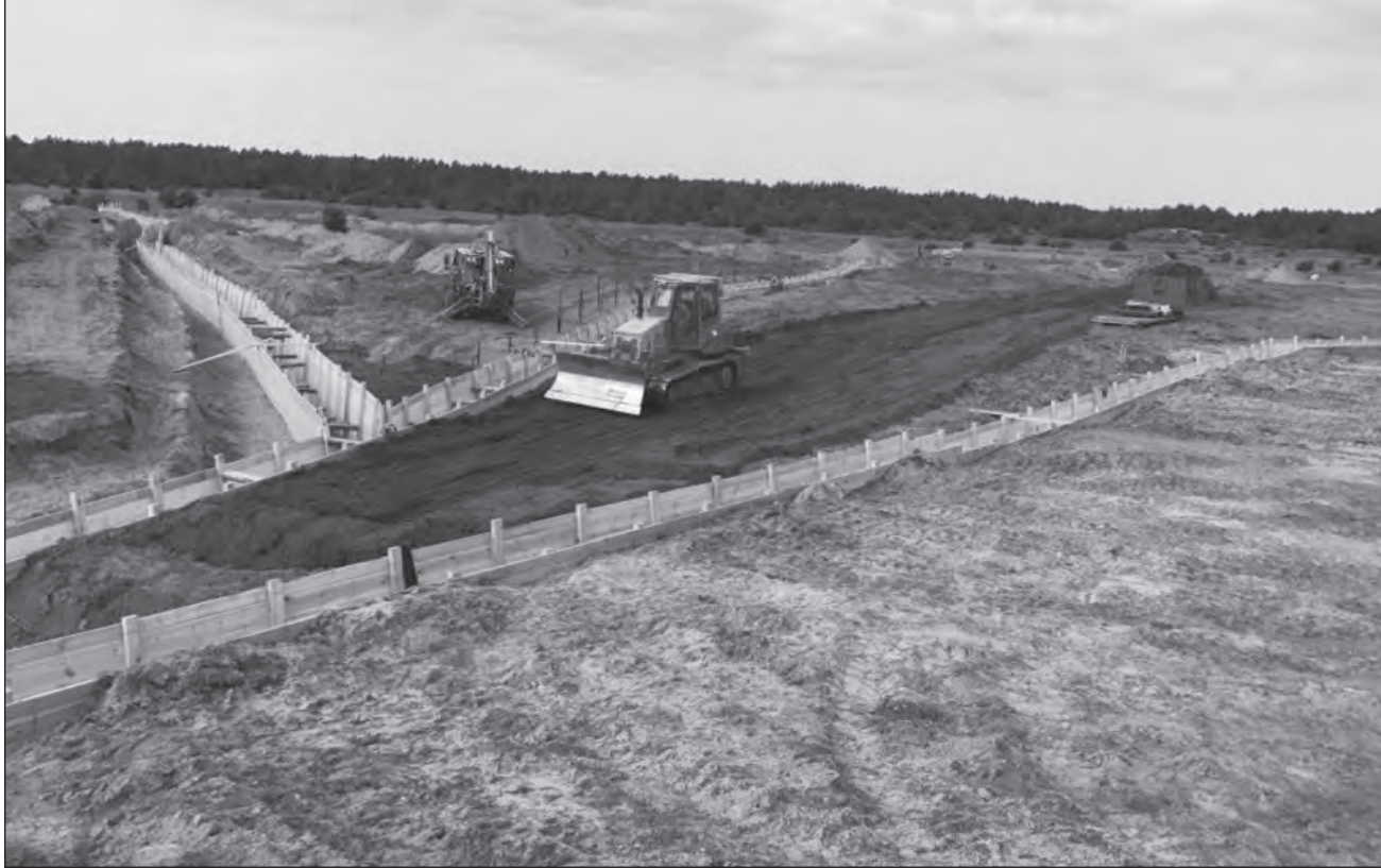
A bulldozer is used to backfill after anchoring.
