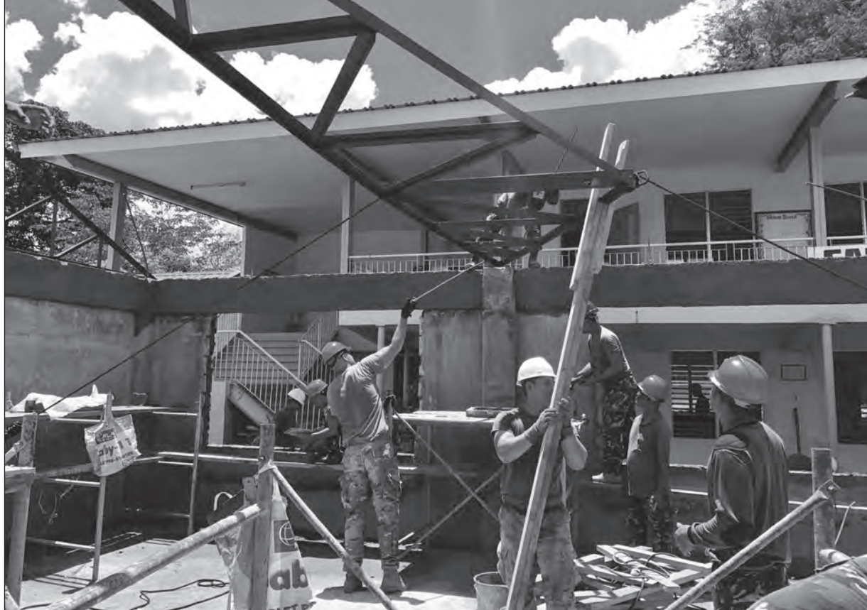
523d Soldiers and host nation counterparts manually hoist a metal truss for the roof system.
