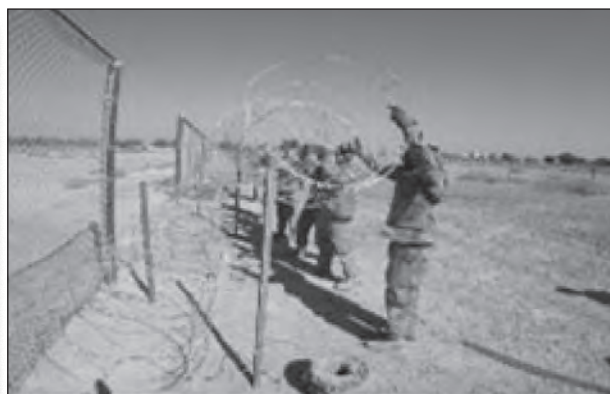
Installation of temporary perimeter fencing to secure the expansion area
