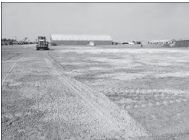
Grading of the expansion area to allow follow-on occupation
