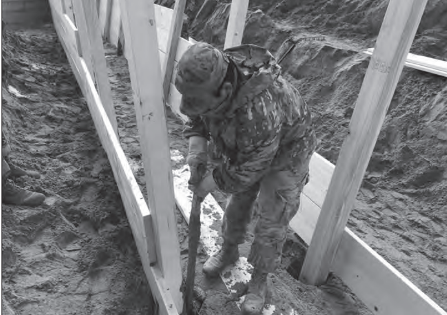
Sapper sifting concrete in the trench.
