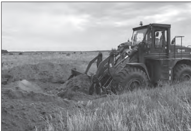
Polish engineers construct a vehicle fighting position.
