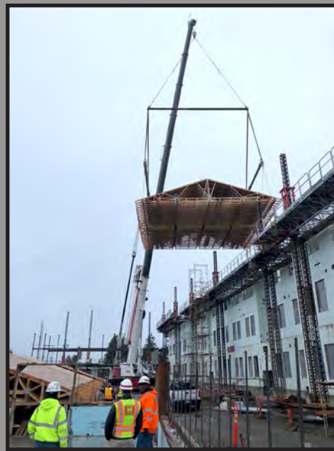
A crane hoists finished sections of roof onto the newly constructed USACE barracks project at Joint Base Lewis-McChord.
