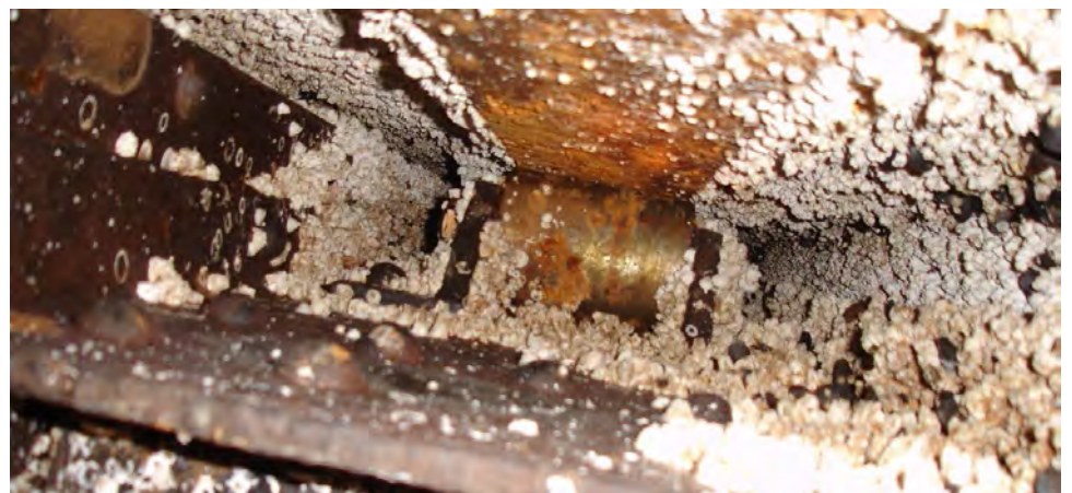
(Top left) Photo of valve gates taken in 1916. (Top right) Original valve gate blueprints. (Below) Barnacle-encrusted rollers on the downstream gates. The rollers are located on the sides of the valve gates.
