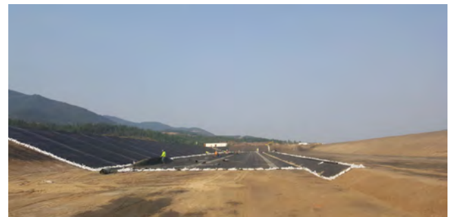
Workers install a geomembrane liner system within one of the triple cells at the newly constructed 110,000 cubic yard sludge impoundment area. (Photo by Greg Zoeller)
