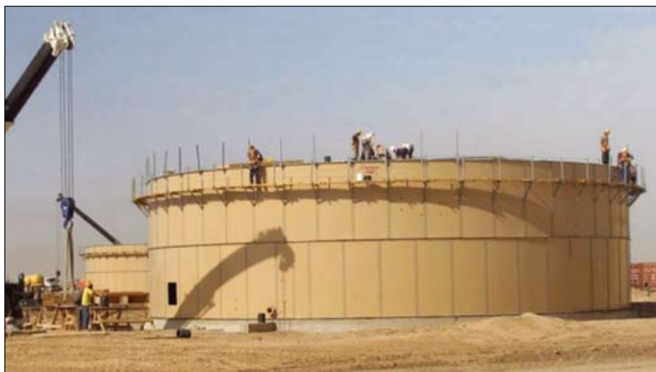
Contractors work on one of the diesel tanks at Contingency Operating Base Speicher Sept. 28, 2008. Sustainers monitored the completion of the $16 million fuel farm construction project, the second “steel-bolted-tank” fuel farm to be operational in theater, replacing the current conventional berm fuel farm. The project will provide COB Speicher an improved facility to issue and receive bulk fuel, to units throughout northern Iraq.
