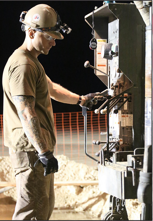
U.S. Navy Construction Mechanic 1st Class Aaron Wymore circulates drilling fluid at the bottom of a bore hole during water well drilling operations in Riohacha, Colombia, Sept. 1. (U.S. Army photo by Staff Sgt. Kalie Frantz)
