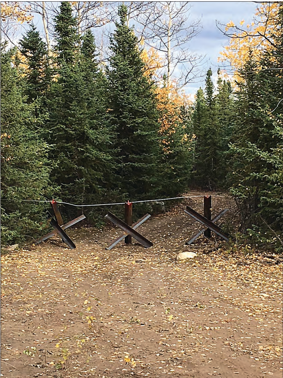
Angle iron, welded into self-supporting barrier stands called hedgehog barriers, are tipped in red paint and connected by steel cables to create a undeniable statement of do not pass. These barriers provide both a visible and physical barricade to protect and warn of culturally sensitive sites on military training lands. (Photo courtesy Fort Wainwright Cultural Resources)
