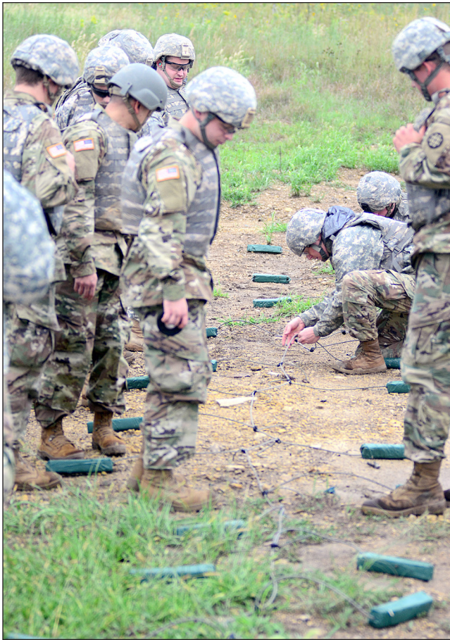
Members of 1st Platoon, 1141st Engineer Company, 203rd Engineer Battalion, 35th Engineer Division, Missouri Army National Guard, inspect their chain of C4 during their familiarization exercise Sept. 7 at Range 52. The 25 groups of C4 each had two-pounds bundled together with detonation cord secured between the two blocks and were set two-feet apart to represent setting off a simulated minefield.
