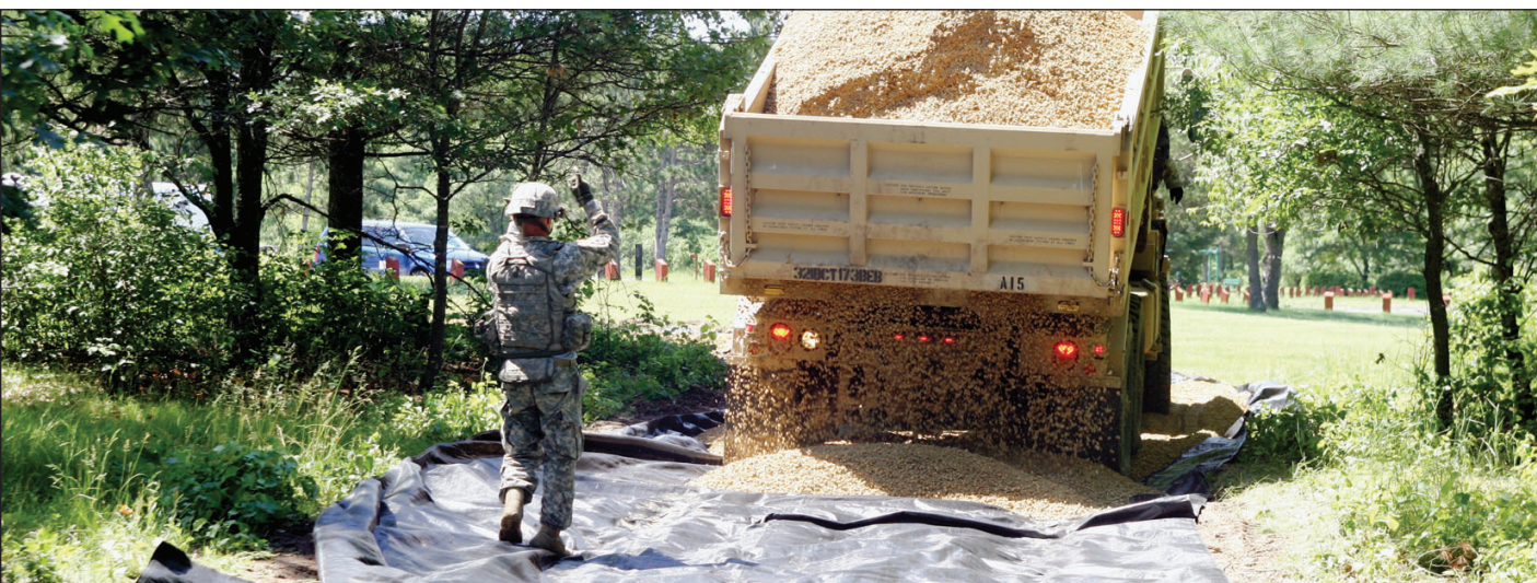
A Soldier guides a dump-truck driver for gravel placement on the road to the new group campsite.
