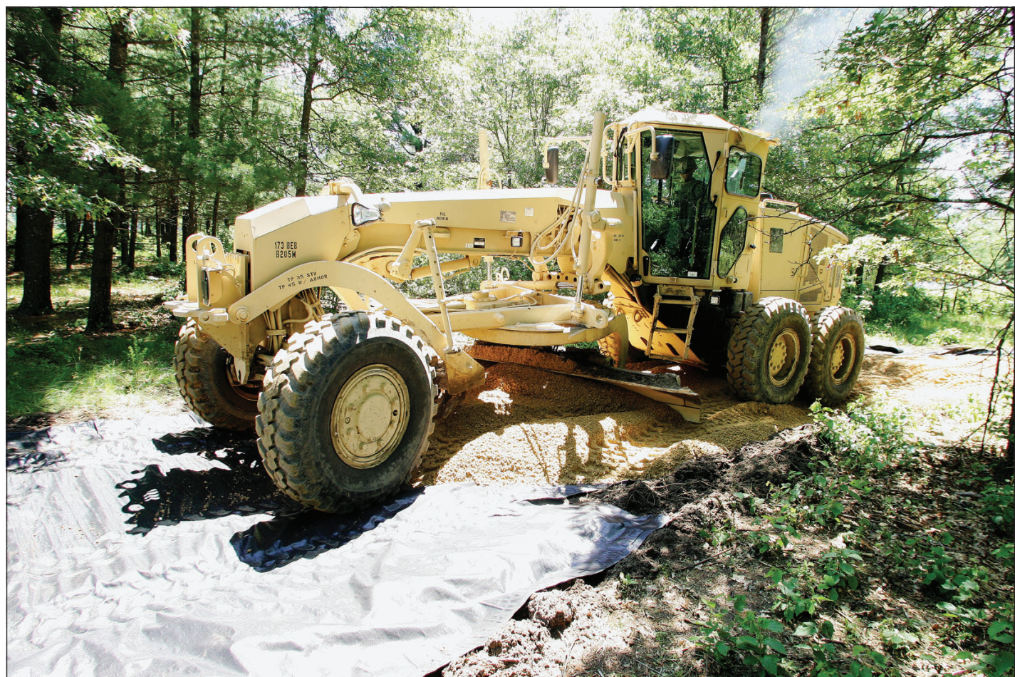
Sgt. Nick Bergman with the 173rd Brigade Engineer Battalion of Onalaska, Wis., operates a grader to spread gravel on a road June 16 at Fort McCoy's Pine View Campground.
