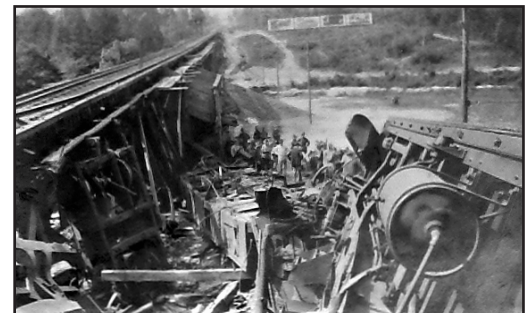
Original photo showing the extent of the damage where the two cars left the tracks. (Courtesy Photo)
