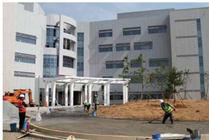
Current construction in progress
