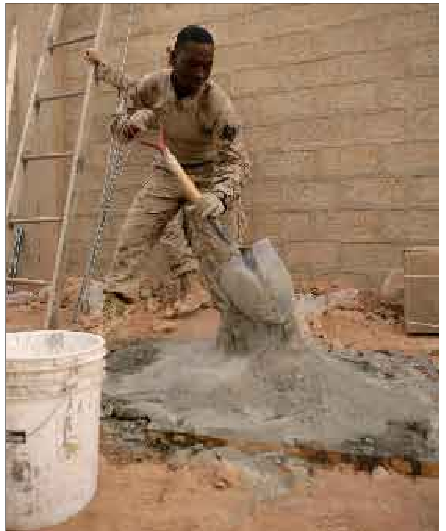
Lance Cpl. Tremayne Baker, a combat engineer from Chicago, with 9th Engineer Support Battalion mixes concrete during final construction in Qasr Amij, Iraq on Oct. 24. The Marines with 9th ESB are working on the facilities for a military transition team operating in the area. Photo by Cpl. James D. Wilkins
