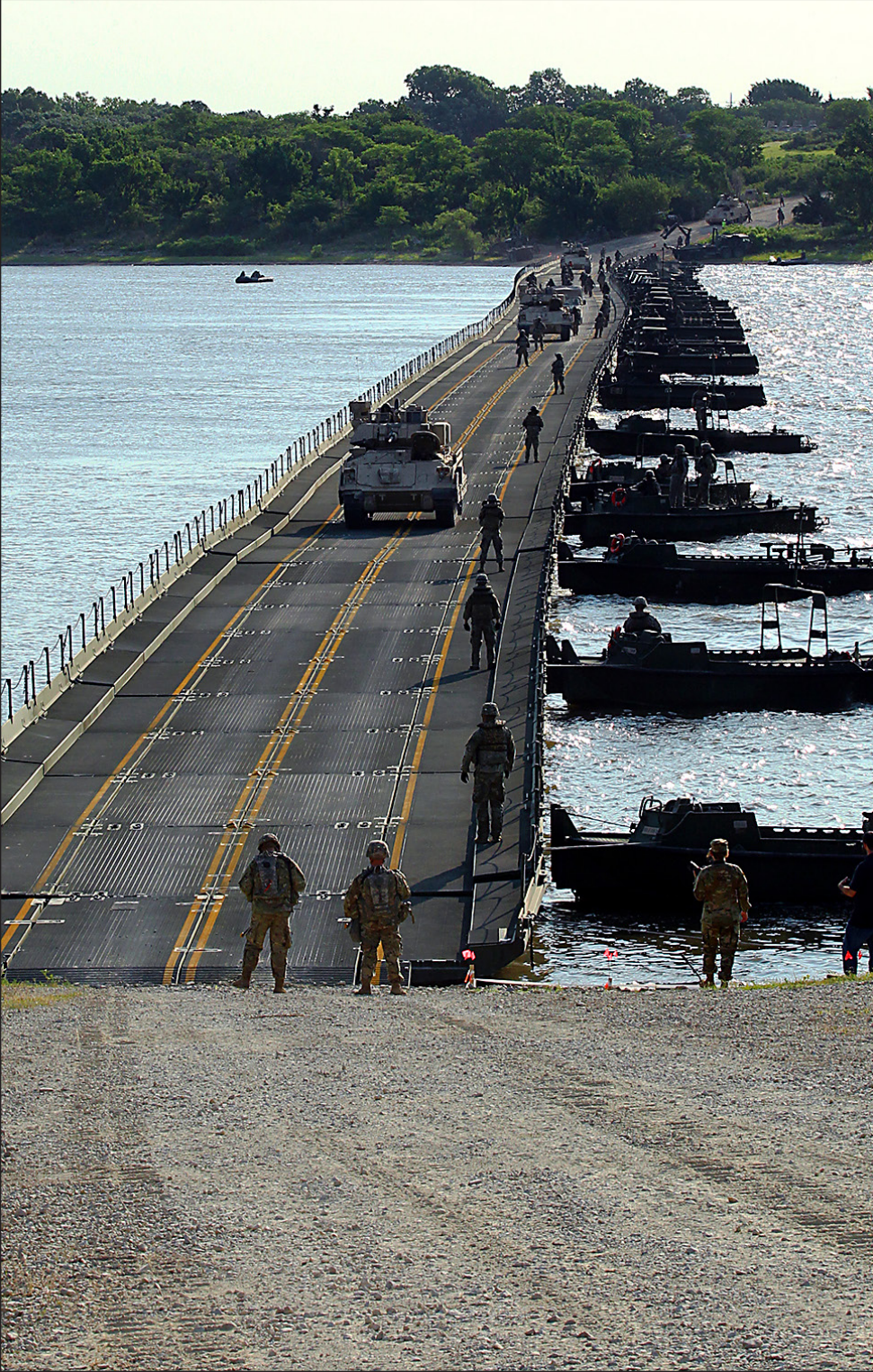
Chad L. Simon | 1st Inf. Div. Public Affairs Bradley Fighting Vehicles and M1A2 Abrams tanks with 1st Battalion, 16th Infantry Regiment, 1st Armored Brigade Combat Team, 1st Infantry Division, cross a temporary, floating bridge at Milford Lake, Kansas, June 15 during training exercise Gauntlet. The 600-meter bridge was constructed by three active-duty Mobile-Role Bridge Companies from throughout the U.S. and a National Guard MRBC from Louisiana.
