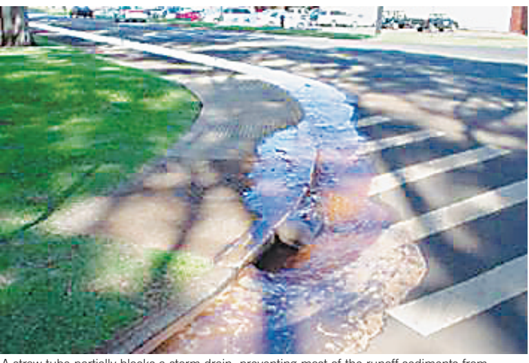
A straw tube partially blocks a storm drain, preventing most of the runoff sediments from reaching local streams and bays. Sediment is classified as a pollutant by the State of Hawaii.
