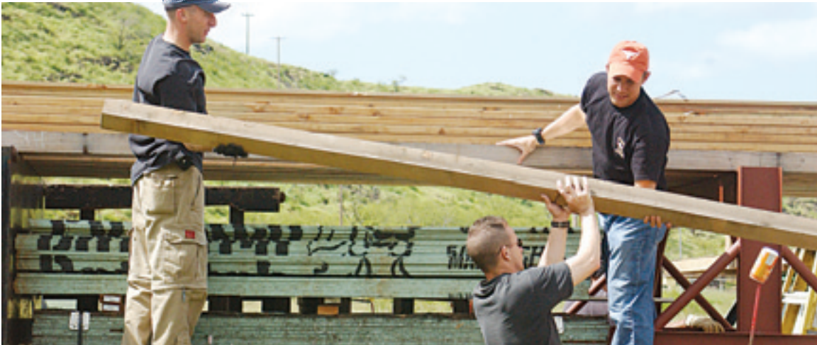
From left, Staff Sgt. Adam Grew, Sgt. James Jeffcoat and Staff Sgt. Carl Holst unload lumber at the Habitat for Humanity house by they will use for construction. Six other Wolfhounds contributed to building a house for a family who had been living out of a makeshift garage.
