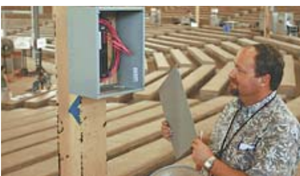
John Draude, principle deputy, information management division, Tripler Army Medical Center, examines one of several boxes the 30th Signal Battalion installed in Conroy Bowl, the primary Soldier Readiness Processing (SRP) and Reverse SRP site on Schofield Barracks. The boxes extend data and network services from the communications room and serve as distribution points for network and telephone support services.
