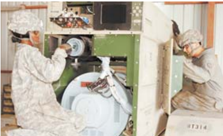
Pfc. Tammy Gallaher (left) and Spc. Michael Boyle, both power generation equipment repair specialists, Headquarters Support Company, 209th Aviation Support Battalion, 25th Combat Aviation Brigade, repair and service a 60-kilowatt generator at Contingency Operating Base Speicher, Iraq, Oct. 30.
