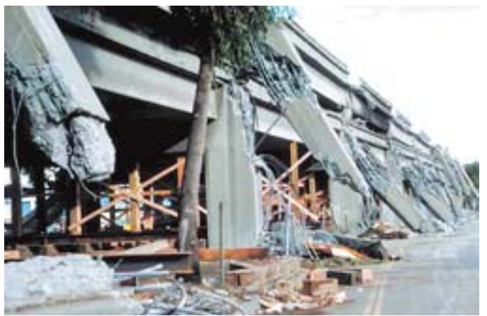
H.G. Wilshire | U.S. Geological Survey The support-columns of the upper deck of the Cypress viaduct, Oakland, Calif., failed and collapsed after the Loma Prieta earthquake, Oct. 17, 1989.
