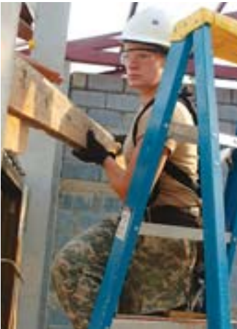
Pfc. Michelle Almeida sets a form in place above a door in the new classroom facility.
