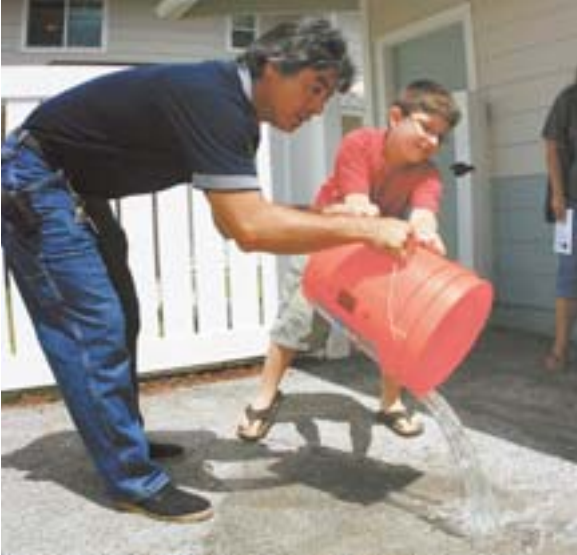
Hamilton resident William Brown gets some help from AHFH maintenance tech Baron Loftin to demonstrate how quickly permeable concrete — one of many LEED for Gold home features — absorbs water.
