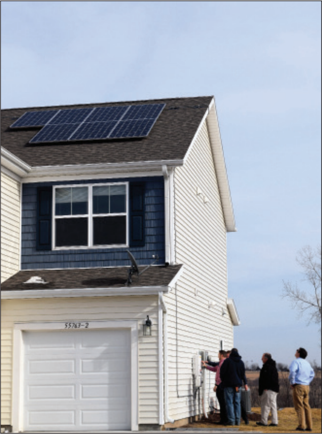
Corvias staff checks out the power inverter that converts direct current to alternating current from the first running solar panels in Fort Riley at the Warner Peterson neighborhood Feb. 8. By October, there will be about 1,200 solar panels installed on residential rooftops on post.
