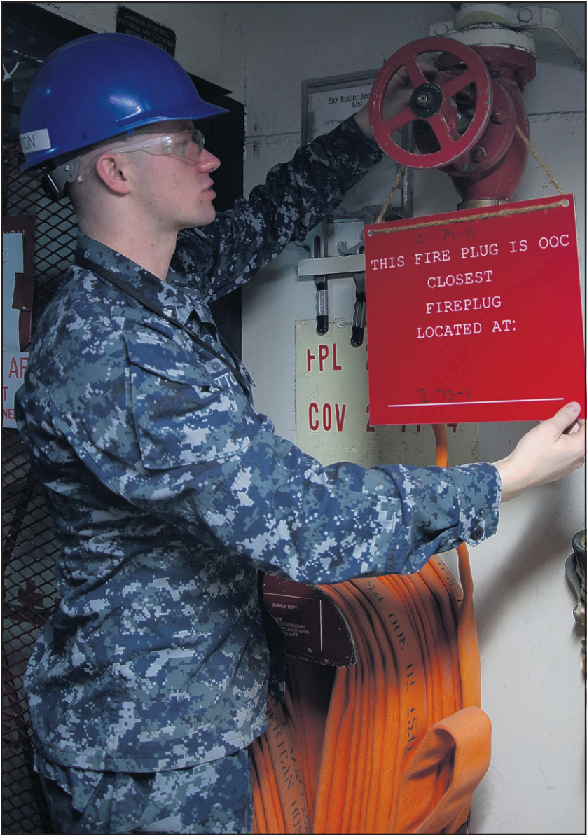
MCSN Julie N. Vujevich Damage Controlman 3rd Class Carter Gratton places a sign on an out of service fire plug on the ship. The aircraft carrier USS George Washington (CVN 73) is undergoing a refueling and complex overhaul (RCOH) at Newport News Shipyard.
