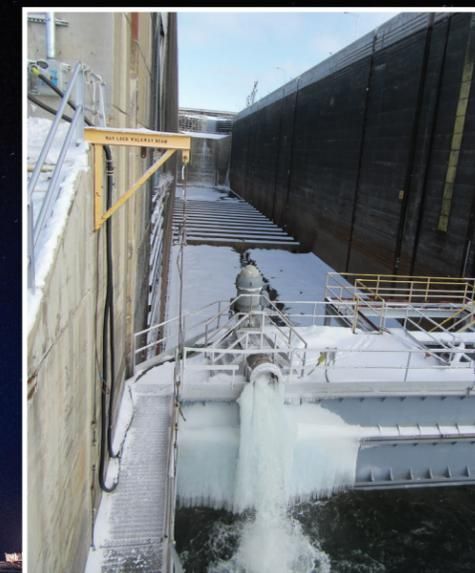
Right, above : Ice Harbor Lock and Dam upgraded critical components of the operating machinery for the downstream gate. Right and below: Replacement of the remaining original gudgeon arm, linkage and the pintle assembly for both gate leaves.
