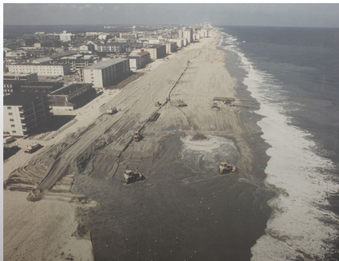
SAND IS PUMPED ONTO THE BEACH AT OCEAN CITY IN 1991 AS PART OF INITIAL CONSTRUCTION OF THE BEACH BERM AND DUNE THAT ARE PARTS OF THE COASTAL STORM RISK MANAGEMENT PROJECT THERE.
