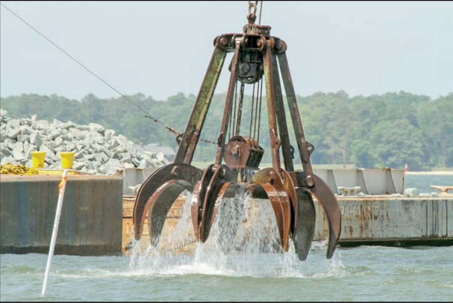
With the help of global positioning satellites, granite rock is methodically placed in the Piankatank River near Gwynn's Island in Mathews County, Va. The rock is the basis for the newest 25-acre oyster reef in the Chesapeake Bay Watershed.
