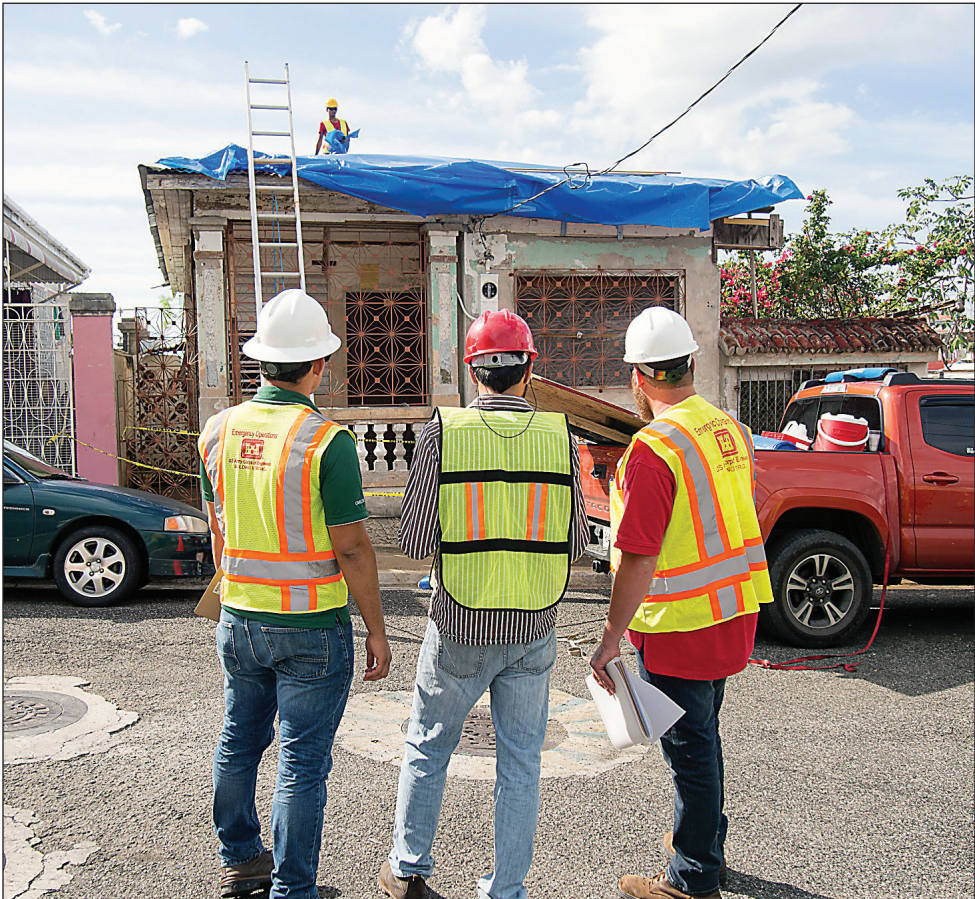
Eric Jones | U.S. ARMY Andrew Lorenz, right, a Quality Assurance specialist with the U.S. Army Corps of Engineers, works with contractors to make a material adjustment at a home receiving a temporary blue roof in Mayagüez, Puerto Rico, Dec. 30.
