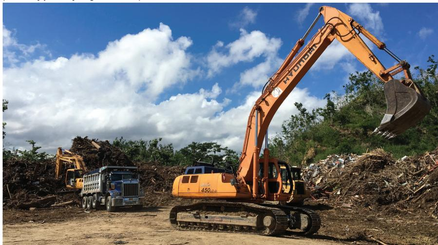
**Left: An excavator repositions for operations unloading and loading trucks at the Trujillo Alta temporary disposal site. Temporary sites serve as municipal collection points for woody debris before it's reduced to mulch or transferred to another location for permanent deposition (mulch recycling site or landfill).** *(U.S. Army photo by Keith Hyde)*
