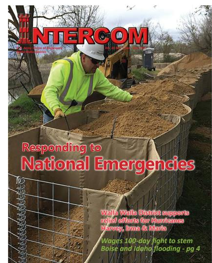
**Corps builds levee to prevent Boise River flooding near Eagle Island, Idaho.** *US Army Corps of Engineers photo)*
