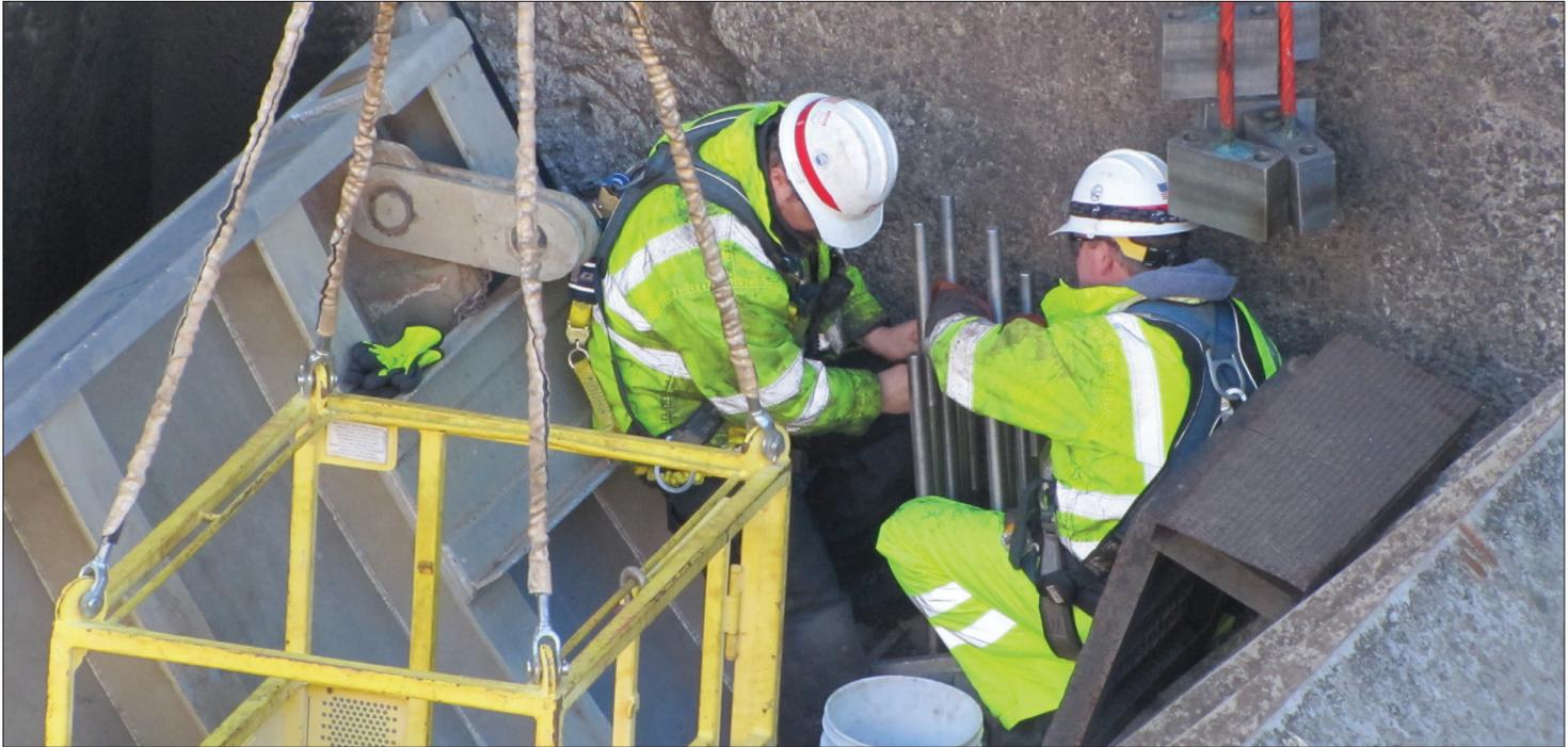
**Mechanical crew lead, Matt Dinotto, oversaw mechanics Dave Sears and Frank Hudson as they wielded the giant gear used to turn the cable drum which operates the massive 86 ton, 27 foot high by 86 foot long upstream gate.**
