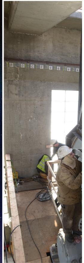
**Right, above :** Ice Harbor Lock and Dam upgraded critical components of the operating machinery for the downstream gate. **Right and below:** Replacement of the remaining original gudgeon arm, linkage and the pintle assembly for both gate leaves.
