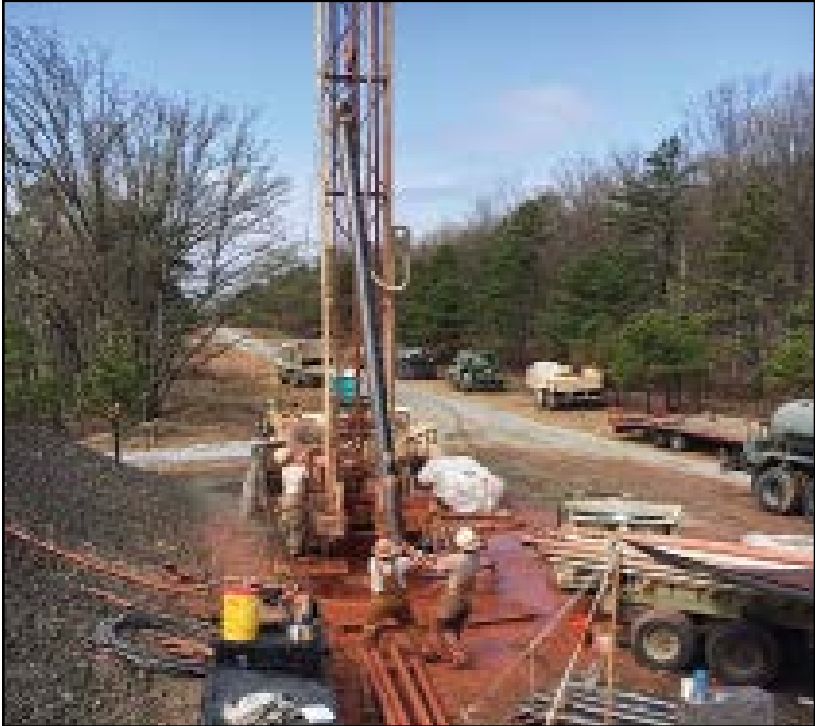
Members of the 247th Engineer Detachment, CTARNG conduct drilling operations at Fort Indiantown Gap, Pennsylvania, April 20, 2017. The unit spent its two-week annual training period at FIG constructing the 300-foot well that will be utilized by base firefighting equipment in the event of a brush fire. This is the third well that the 247th has drilled at FIG in the last three years. (Photo courtesy of the 247th Engineer Detachment, CTARNG)
