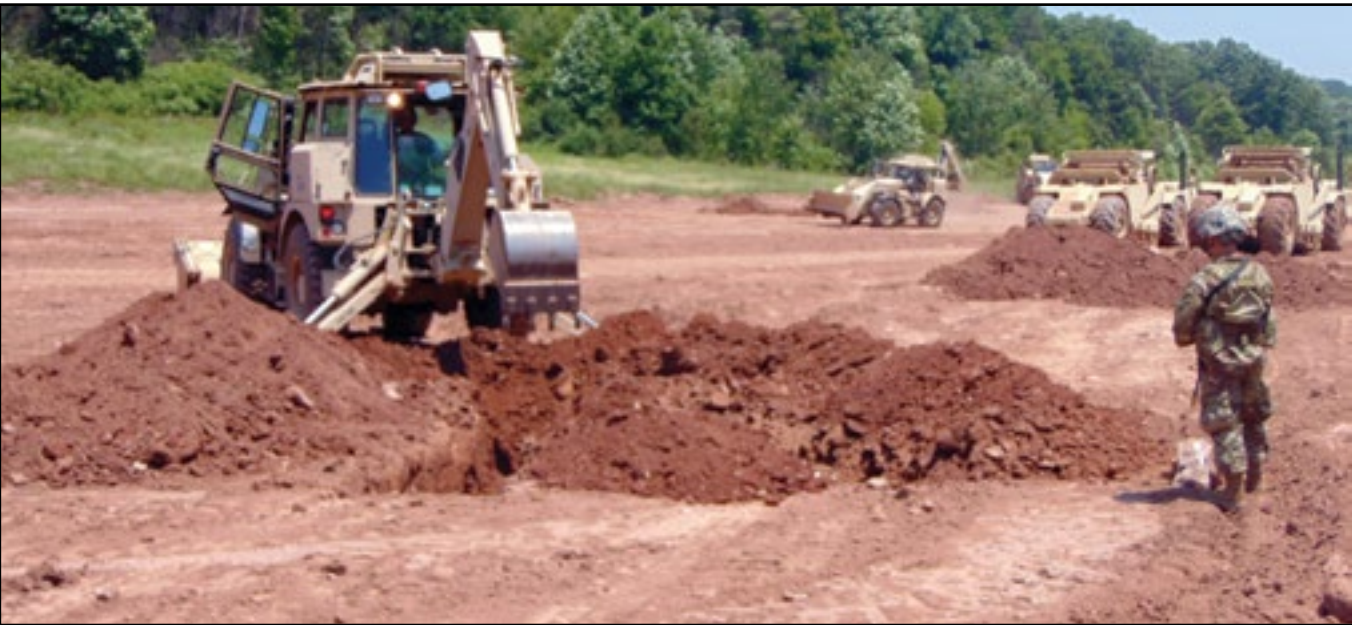
Members of the 248th Engineer Company train on various pieces of heavy equipment at Fort Indiantown Gap, Pennsylvania, June 11. Soldiers conducted clearing and grubbing operations, preparing an area for a new artillery firing point. (Photo by Sgt. Victoria Tuttle, 248th Engineer Company, 192nd Engineer Battalion)
