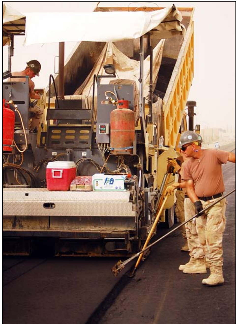
Workers from the NMCB 74 rake fresh asphalt as it comes out of the paving machine. The crew of 'Can Do' Seabees withstood relentless heat to provide a paved loop around Zone Six on Camp Arifjan, Kuwait.
