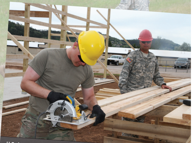
U.S. Army Pfc. John Weischedel and Sgt. Chad Bergen, 155th Engineer Company, South Dakota Army National Guard, trim boards with a circular saw for a storage building on Camp Rapid, Rapid City, June 16. (U.S. Army National Guard photo by Spc. Rebecca Glidden)
