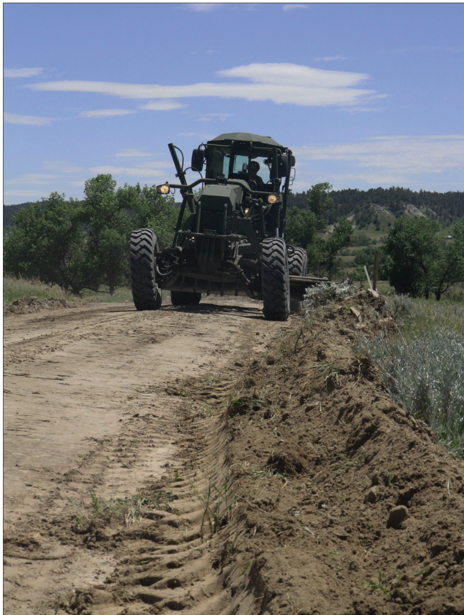
A Soldier with the 842nd Engineer Company uses a grader to level off the edges of the road created by a roller along JB Pass Road in Gallatin National Forest, June 15. (U.S. Army National Guard photo by Staff Sgt. Rachel Korzeniewski)
