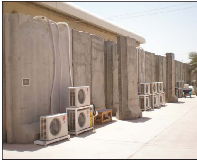
Photo provided by FOB Blackhawk Mayoral Cell New "split" air conditioner units provide cooler air to the FOB's tenants and use less energy than previous models.
