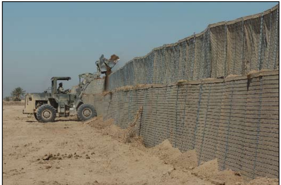
Photo by Sgt. Jason Stadel A front-end loader from the 535th Engineer Company fills Hesco barriers at Patrol Base Vanderhorn March 6.
