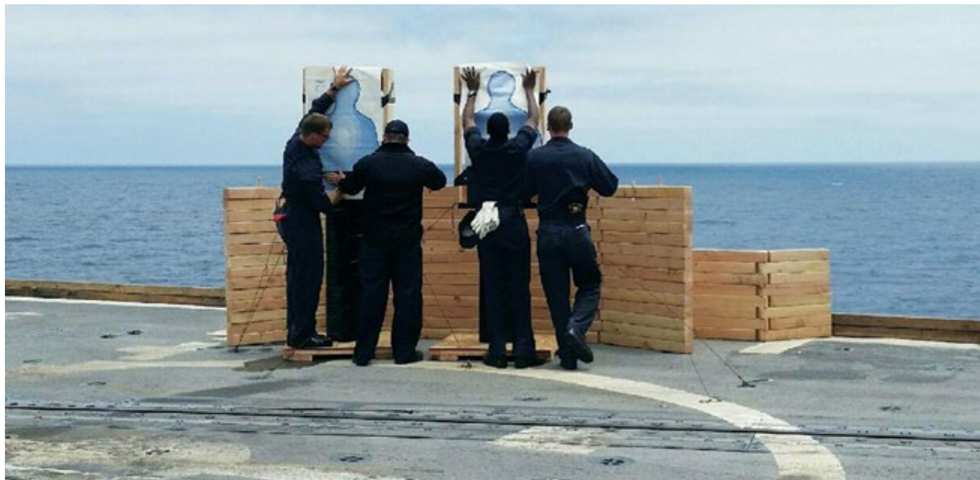
USS CAPE ST. GEORGE (CG 71) crew installs flight-deck range protective barriers made of pressure-treated wood and galvanized piping.
