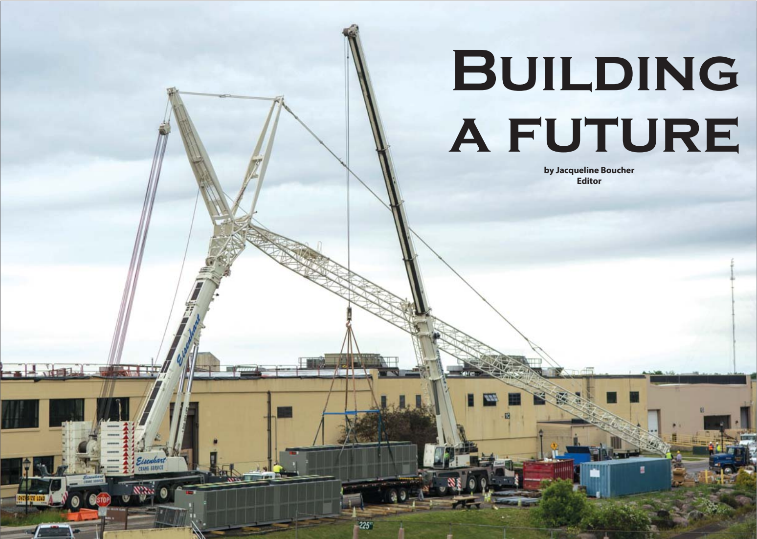
One of several chillers that will offer energy efficient solutions for an industrial cooling application is lifted onto the roof of Building 1A with a 550-ton capacity crane. (Photo by Jim Lentz)
