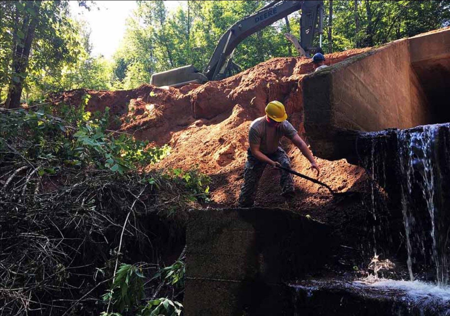
Members of the 229th Engineer Company, including Sgt. Chad Buchen (foreground), backfill a washed-out culvert along Eade Road in Ashland County, Wis., as part of flood recovery operations. Wisconsin National Guard photo by Sgt. Kimberly Miannecki
