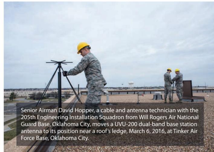
Senior Airman David Hopper, a cable and antenna technician with the 205th Engineering Installation Squadron from Will Rogers Air National Guard Base, Oklahoma City, moves a UVU-200 dual-band base station antenna to its position near a roof's ledge, March 6, 2016, at Tinker Air Force Base, Oklahoma City.
