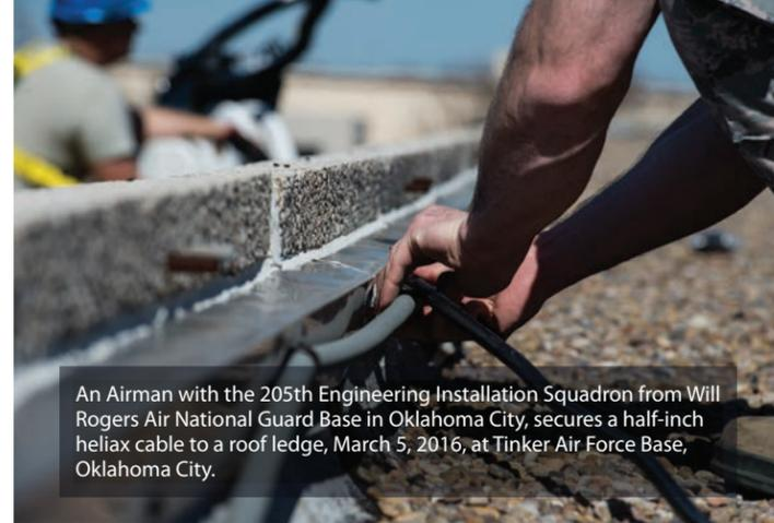
An Airman with the 205th Engineering Installation Squadron from Will Rogers Air National Guard Base in Oklahoma City, secures a half-inch heliex cable to a roof ledge, March 5, 2016, at Tinker Air Force Base, Oklahoma City.
