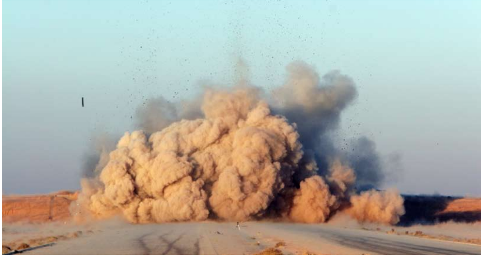
Debris is sent flying into the air as Bridge 18 is demolished by the Marines of Company C, 1st Combat Engineer Battalion, Regimental Combat Team 2, Dec. 3. The Marines used 2,080 sticks of C-4 explosive to destroy the bridge.
