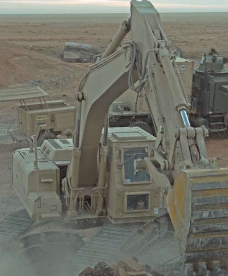
A Co. C heavy equipment operator kicks up dust as he uses an excavator to tear at pieces of the demolished Bridge 18 Dec. 3. The bridge was destroyed to make it safe for large vehicles to pass underneath.
