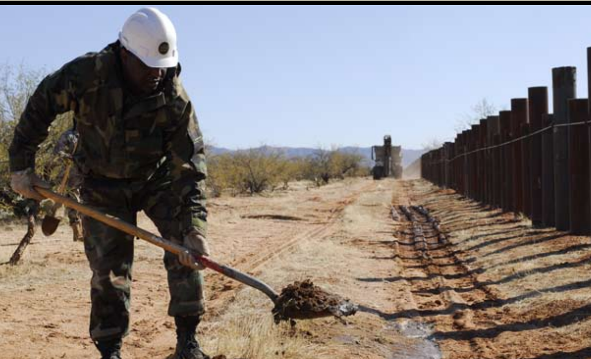
Staff Sgt. Gary Patterson of the Georgia Air National Guard's 283rd Combat Communications Squadron, deployed to Operation Jump Start – Arizona's Task Force Diamondback, shovels dirt into the hollow permanent vehicle barriers in San Miguel, Ariz.
