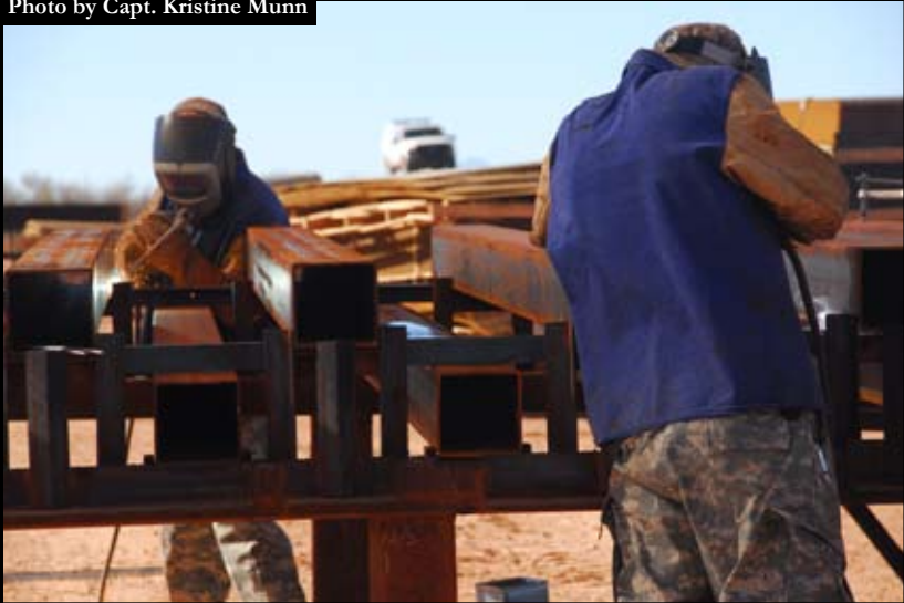
In the background, a Border Patrol agent keeps vigilance over the area while Soldiers with the Michigan Army National Guard assigned to the engineering element of Operation Jump Start, Task Force Diamondback, weld together steel railroad rails which are being recycled to form part of the fence in Douglas, Ariz.
