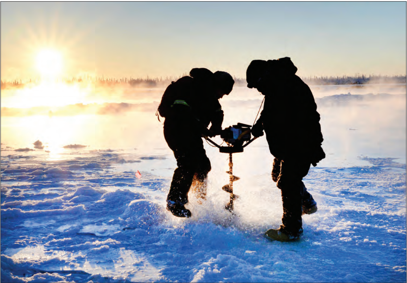
Senior Airman Carlos Aleman, a 354th Civil Engineer Squadron range maintenance technician, uses an auger to drill a hole in the frozen Tanana River with Tech. Sgt. Craig Slaten, the 354th CES noncommissioned officer in charge of service contracts, Dec. 5, in Fairbanks, Alaska. Slaten and Aleman use the auger to drill into the ice, exposing water which will build up the ice and create a stable bridge for transportation of equipment and supplies. (Photo by Airman 1st Class Cassandra Whitman, 354th Fighter Wing Public Affairs)
