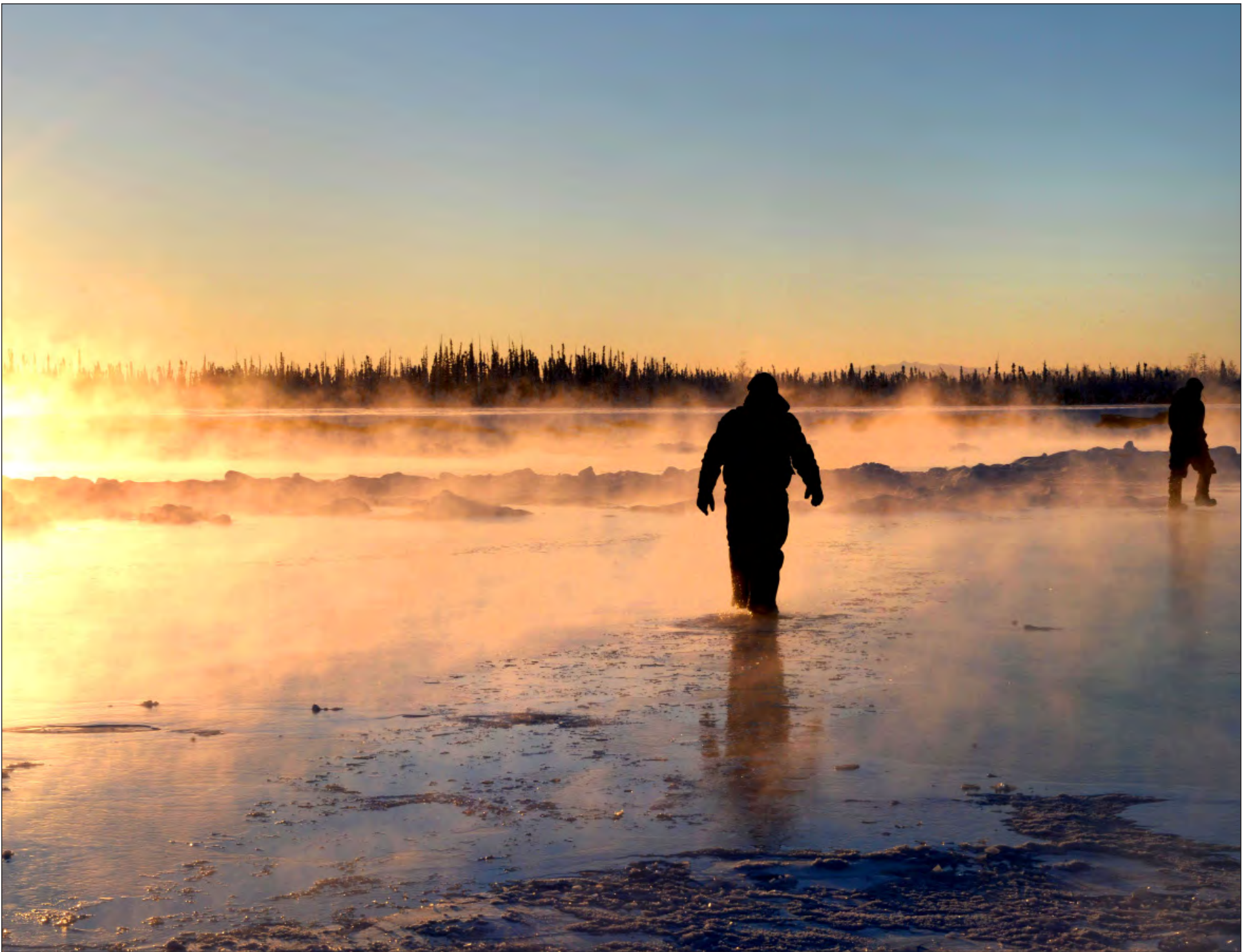
U.S. Air Force Senior Airman Carlos Aleman, a 354th Civil Engineer Squadron range maintenance technician, walks through water as it freezes over existing ice on the Tanana River with Tech. Sgt. Craig Slaten, the 354th CES noncommissioned officer in charge of service contracts, Dec. 5, 2016, in Fairbanks, Alaska. A team of Airmen build up the ice bridge every two years to make transportation of equipment and materials easier for the Airmen and civilians who work at the Blair Lakes Range Maintenance Complex. (Photo by Airman 1st Class Cassandra Whitman, 354th Fighter Wing Public Affairs)
