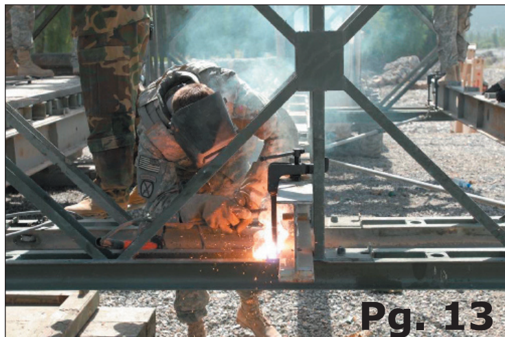
A Soldier from the 70th Engineer Battalion welds pieces of a 110-foot bridge at Jaji, Afghanistan. The bridge will allow Afghans to cross a river and use a prevalent supply route.
