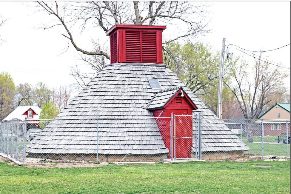
A hand-dug well sits in the center of Seneca City Park on 11th Street. It was dug in 1895, and it is the last visible sign of the original water system installed in 1895. The well is 65 feet deep and 34 feet wide. "It's the widest hand dug well in Kansas," said Darlann Rial, corresponding secretary for the historical society.
