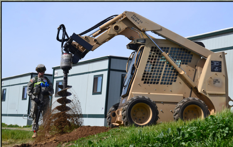
Above: Spc. William Shaw (left) provides safety and ground guides Sgt. Timothy Marler, both with the 389th Engineer Company, while drilling post holes for a stairs project during Combat Support Training Exercise 78-16-01 at Fort Hunter Liggett, Calif. (U.S. Army photo by Sgt. Steffanie Collazo)
