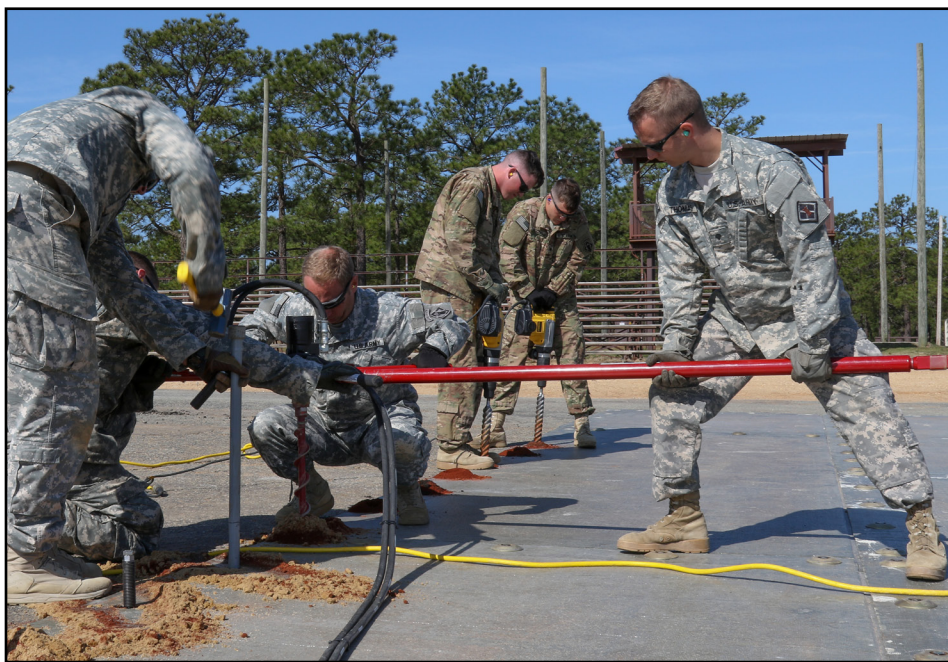
Engineers assigned to the 844th Engineer Battalion drill holes to install a fiberglass polymer matting system during airfield damage repair training on Fort Bragg, N.C., March 8, 2016. For the past three weeks, horizontal construction engineers from throughout the installation observed and demonstrated airfield damage repair techniques on Sicily Drop Zone under the tutelage of the Engineer Research and Development Center. (U.S. Army photo by Staff Sgt. Jason Hull)
